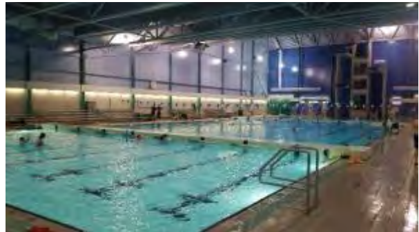
Shallow end bulkhead
