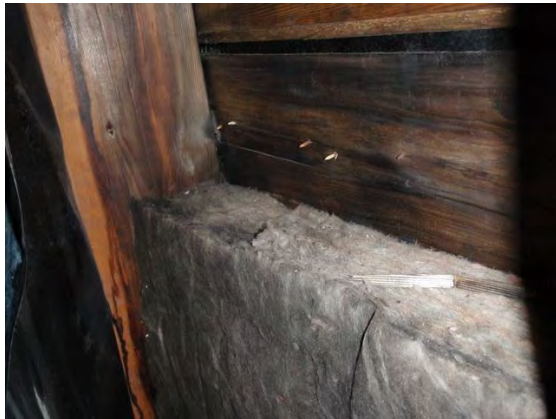
Photo 3, 4: Shows the mansard construction of the east and north walls. Interior polyethylene vapour barrier, 2 X 8 dimensional supports fastened to a structural steel framing, 1 X 8 planking. On the exterior is building paper and cedar shingles. Note the staining of the wood. The shingle fasteners penetrating the planking are corroded from exposure to moisture [chlorine?].
