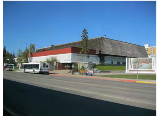
North East Corner
