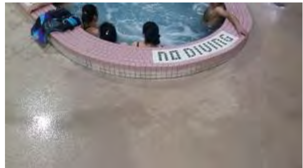
Spa deck plaster
