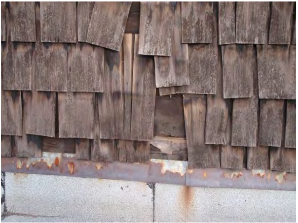
Photo 6, 7: The shingles have come lose and have deteriorated to the point where they are not fastened properly and are not providing the water penetration protection they were designed to provide.
