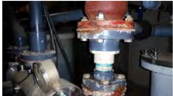
Corroding flanges
