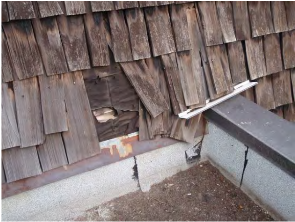
Photo 6, 7: The shingles have come lose and have deteriorated to the point where they are not fastened properly and are not providing the water penetration protection they were designed to provide.
