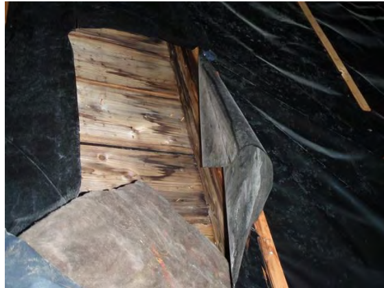
Photo 3, 4: Shows the mansard construction of the east and north walls. Interior polyethylene vapour barrier, 2 X 8 dimensional supports fastened to a structural steel framing, 1 X 8 planking. On the exterior is building paper and cedar shingles. Note the staining of the wood. The shingle fasteners penetrating the planking are corroded from exposure to moisture [chlorine?].
