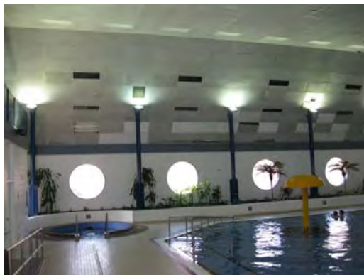
Interior view of 1985 addition
