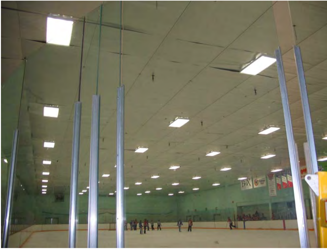
Figure 23: HID to Fluorescent Retrofit
