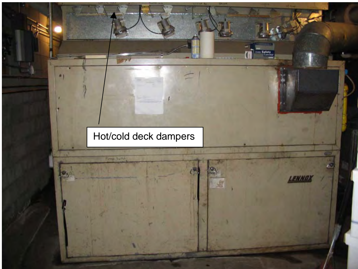
Figure 17: RCMP Multizone System
