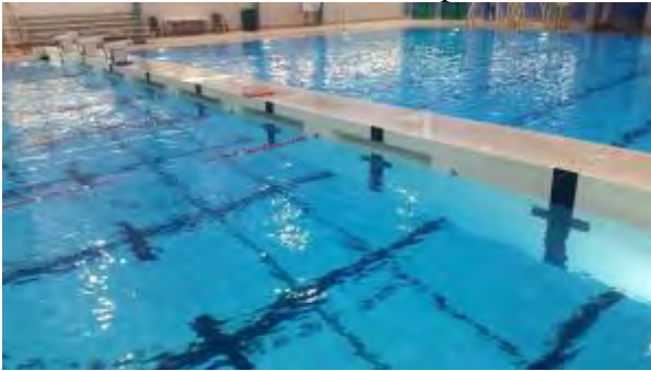
Deep end bulkhead
