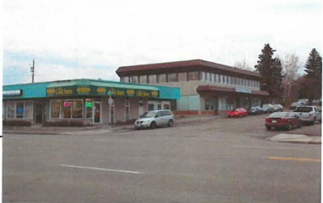
Figure 12: Commercial use on Victoria St. (looking into study area).
