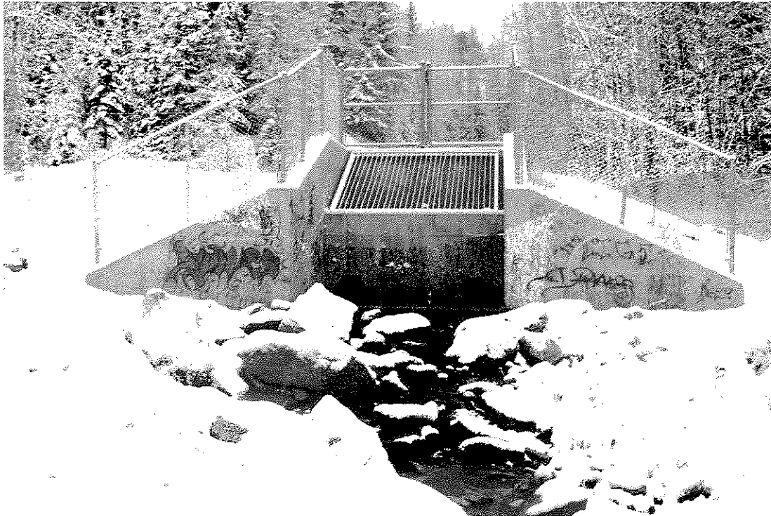
Photograph 7: View of the storm sewer outfall north of Essex Crescent.
