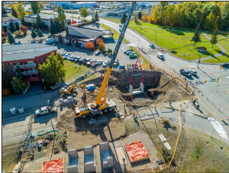
Figure 4: 2018 Winnipeg Street Storm Sewer Repair
