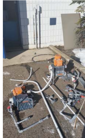
PW 605 Wilson Park West Well Fluoride Injection System Equipment Removed
