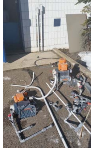
PW 624 College Heights Well Fluoride Injection System Equipment Removed
