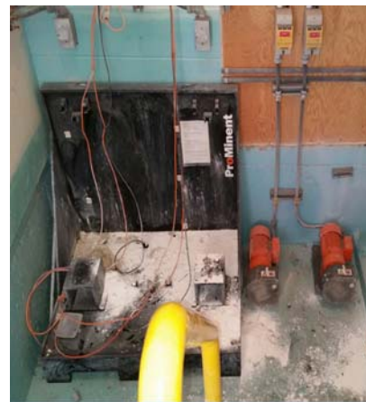
PW 624 College Heights Well Fluoride Injection System Equipment Removed
